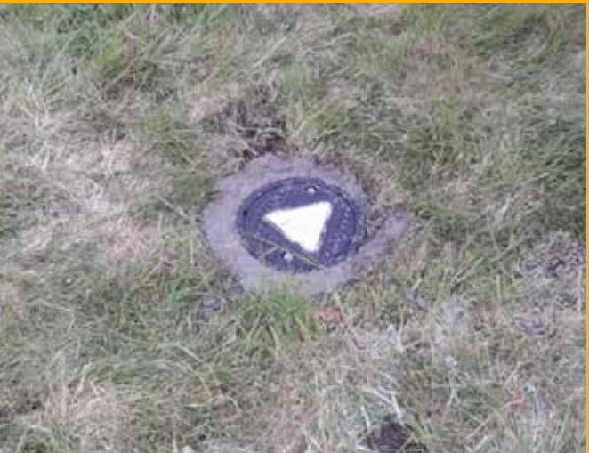
Example of a flush borehole cover
