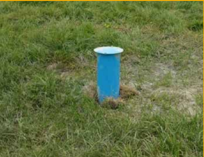
Examples of a raised borehole cover
