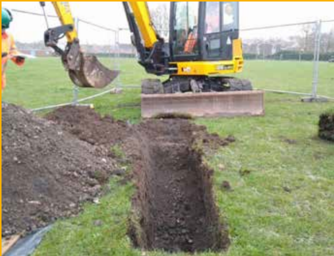
Example of a trial pit on site
