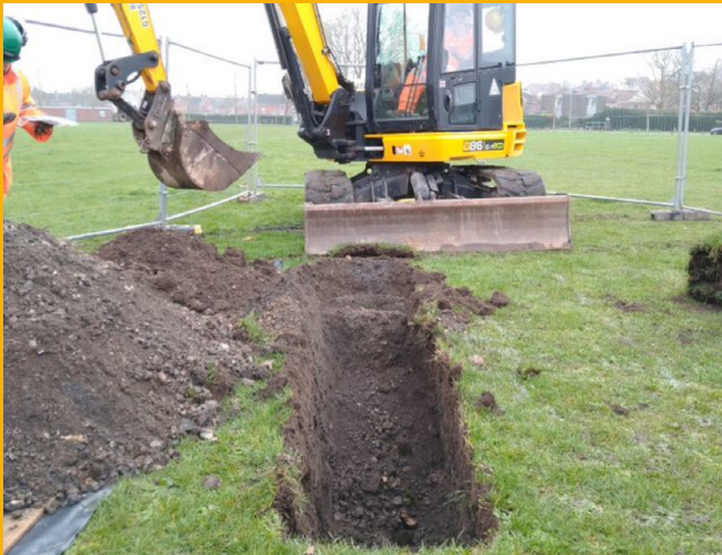
Example of a trial pit on site
