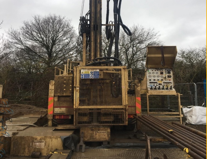
Example of a rotary core rig
