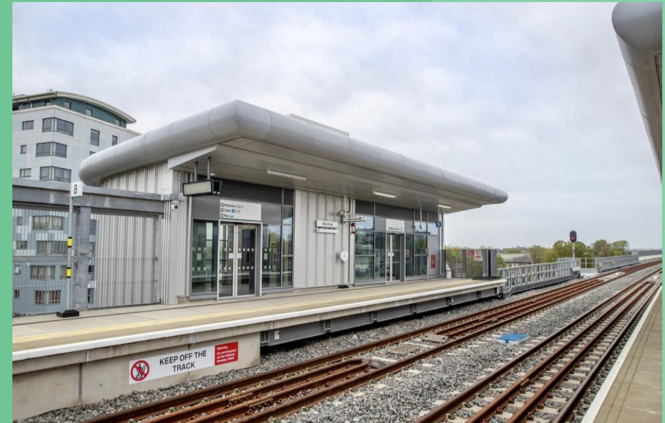
Bletchley station under construction
